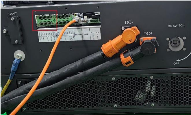
Figure 4- 19 Wiring position of RS485 cable and power cable of PCS
